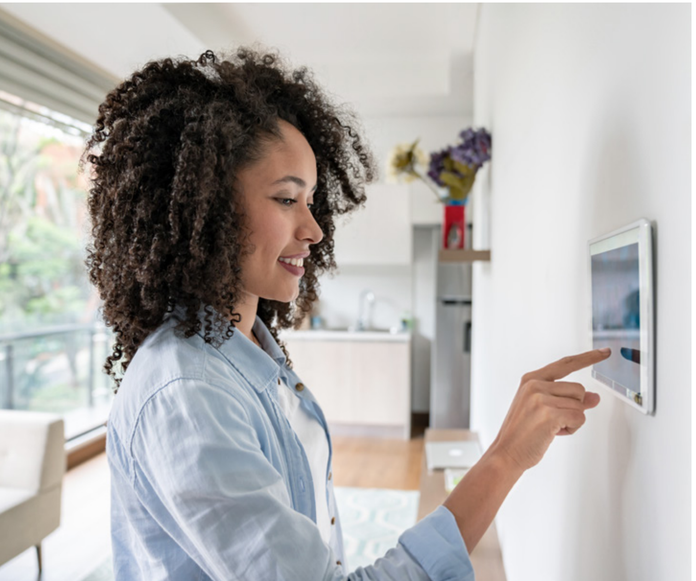
▲ Digital hub for controlling various applications in the apartment.
